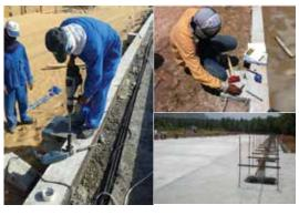
A lighter frame means a lighter concrete base. Each post of the structure stands on a solid concrete block. C-Lines ensures that these concrete blocks adhere fully to local legal codes. The concrete and fast acting chemical anchorage used ensures that C-Lines structures are built fast and most importantly, strong.
